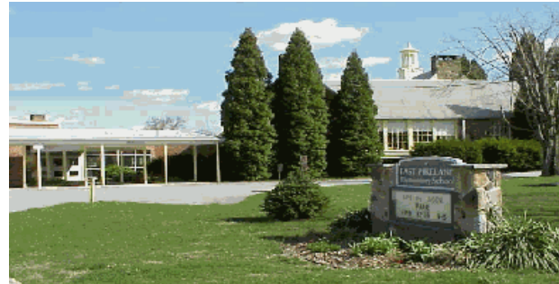
Figure 2: East Pikeland Elementary
